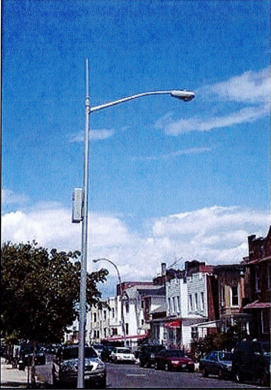
Exhibit 2. The antenna is narrower than, and in scale with the pole. This would be an acceptable design for a cobra-style light fixture.
