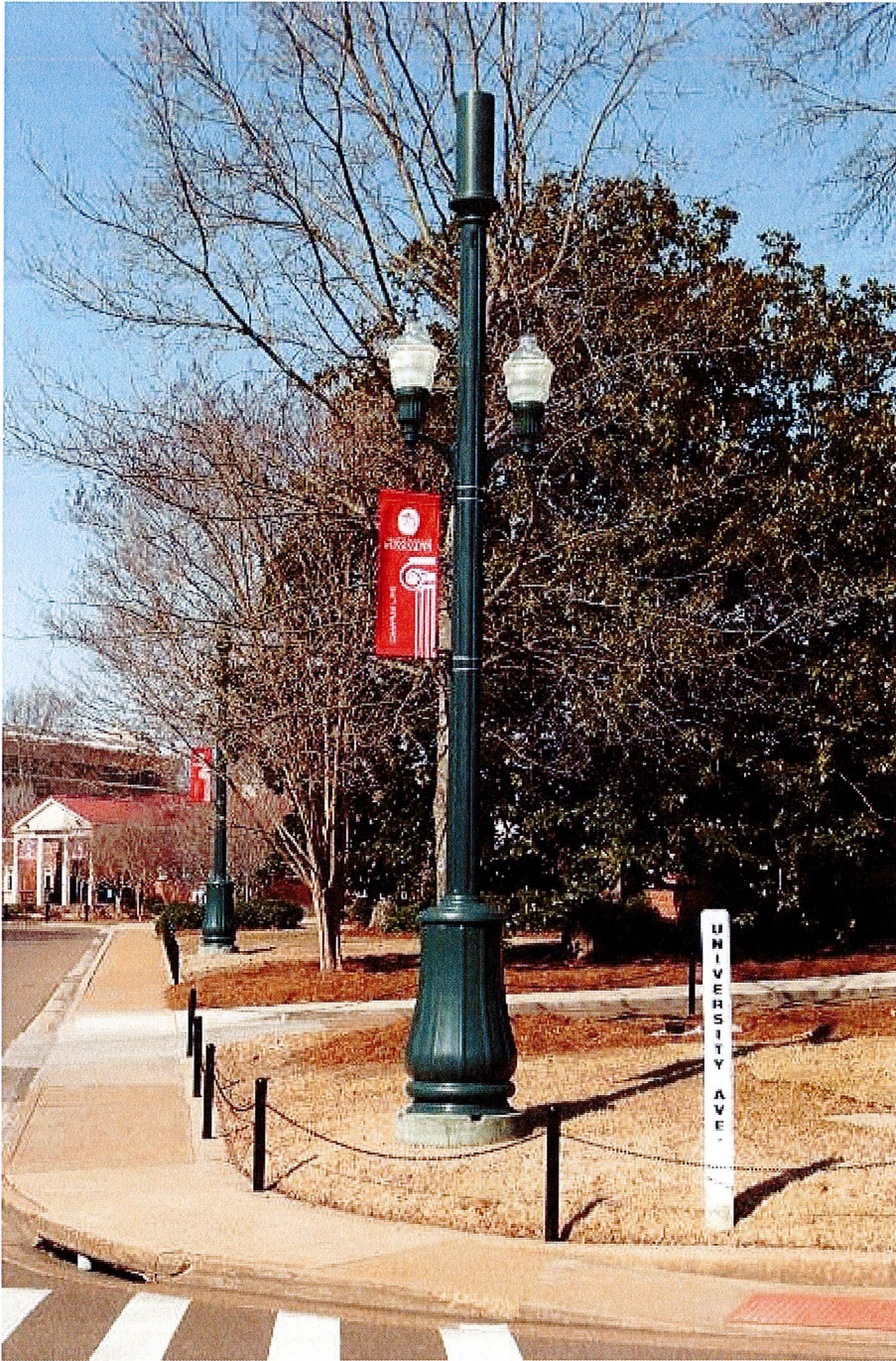
Exhibit 5. This design may be acceptable if consistent with other fixtures in the immediate vicinity. The base is out of scale to the arms and luminaires. In addition, while symmetrical, the pole and antenna extend far above the luminaires, making the design appear vertically out of proportion. Arms and luminaires should be within the top 20% of the pole height. This design is prohibited; however, a similar design may be acceptable with appropriate modifications.
