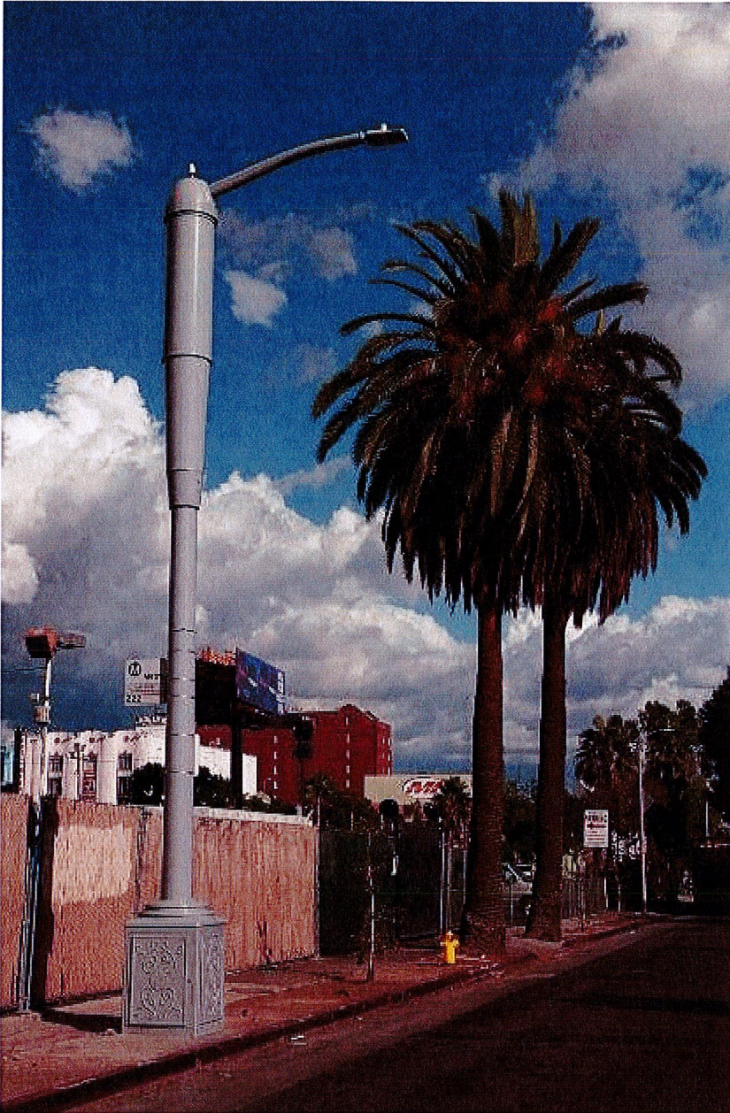
Exhibit 7. The antenna enclosure has a larger diameter than the pole, rendering it insufficiently cloaked. This design is prohibited.
