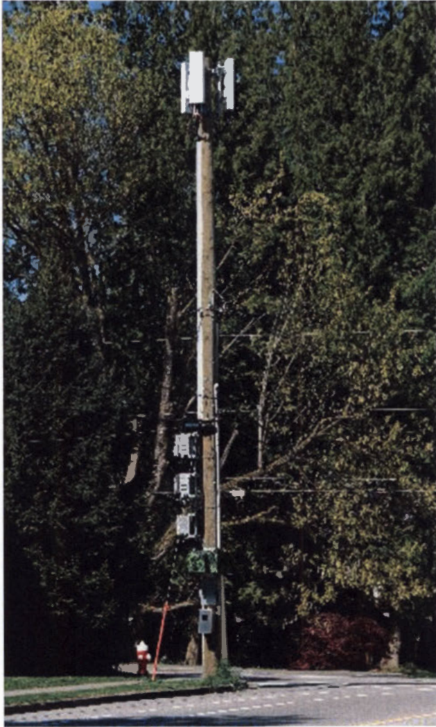
Exhibit 10. Wooden poles are prohibited. The City is transitioning away from wooden poles. In addition, the top-mounted antennas extend on arms away from the pole. This design is prohibited.
