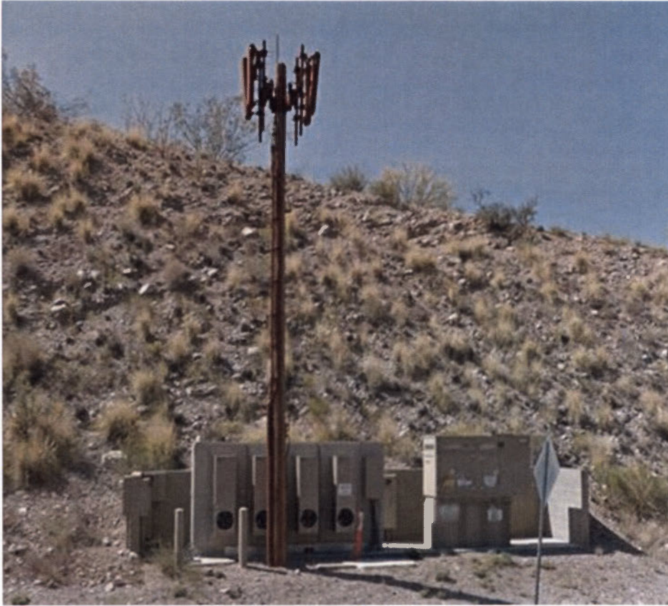
Exhibit 11. Antennas on arms are prohibited.
