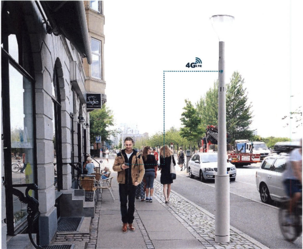
Exhibit 3. An antenna incorporated into, and hidden in the pole of top mounted, pedestrian scaled light may be acceptable if painted black, featured an acorn luminaire, and otherwise substantially resembled the acorn light fixtures already existing in the City. The photo depicts a Philips pole with internal Ericsson antennas.
