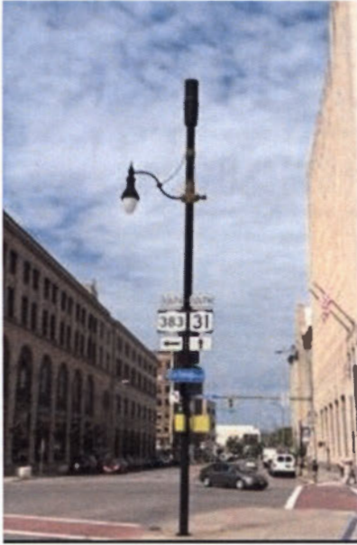
Exhibit 12. The pole lacks a base in scale to the volume of the antenna, which is larger than the diameter of the pole and does not appear to be an original part of the pole. This design would be prohibited.
