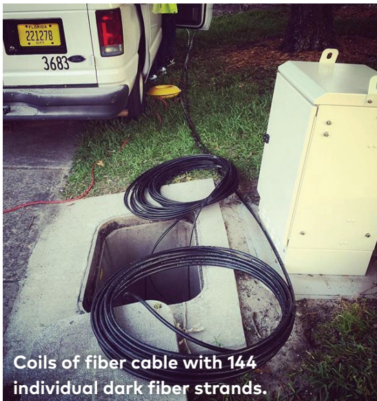
Pulling fiber cable to the main data center in the heart of Winter Haven.
